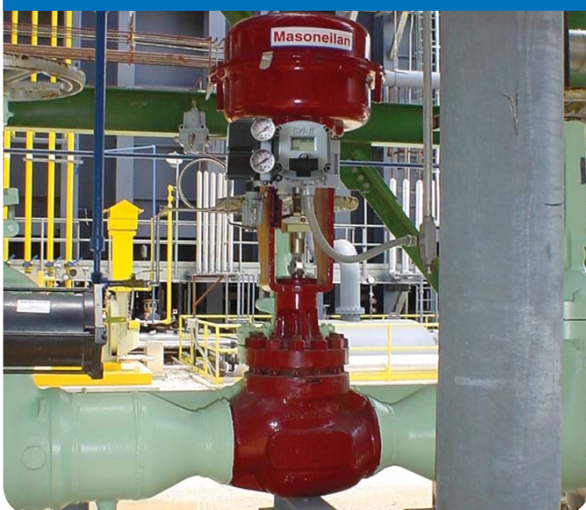
SVI II AP on severe service valve
